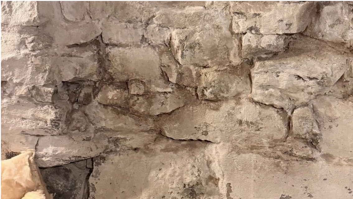
Interior stone foundation conditions reviewed as part of the basement moisture assessment.
